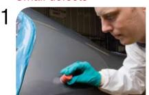
Remove defect using 3M<sup>™</sup> 9 Micron Abrasive Discs 268L (00127).
